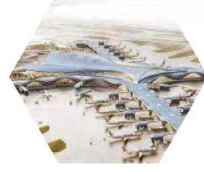
Midfield Terminal Complex Abu Dhabi
